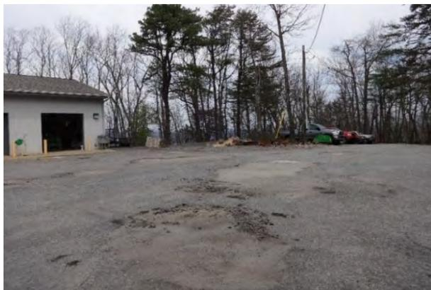
*Existing asphalt needs to be regrading for positive drainage. Need to install asphalt paving, provide staff parking and an area to store materials.*
