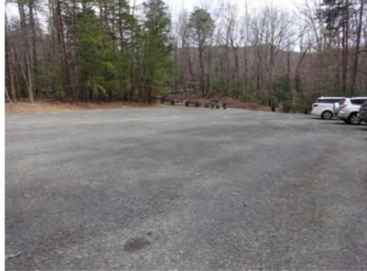
*Parking lot has poor drainage and asphalt is crumbling*
