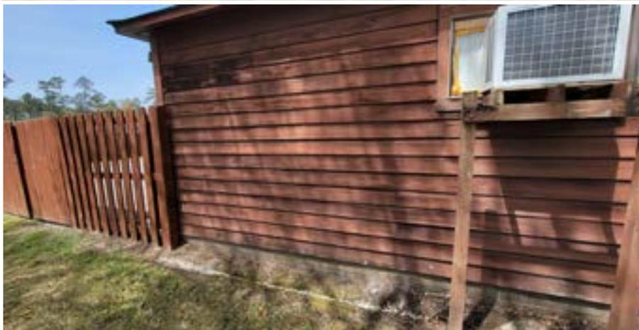
The maintenance building was constructed in 1982. The siding needs to be replaced with sustainable building products.
