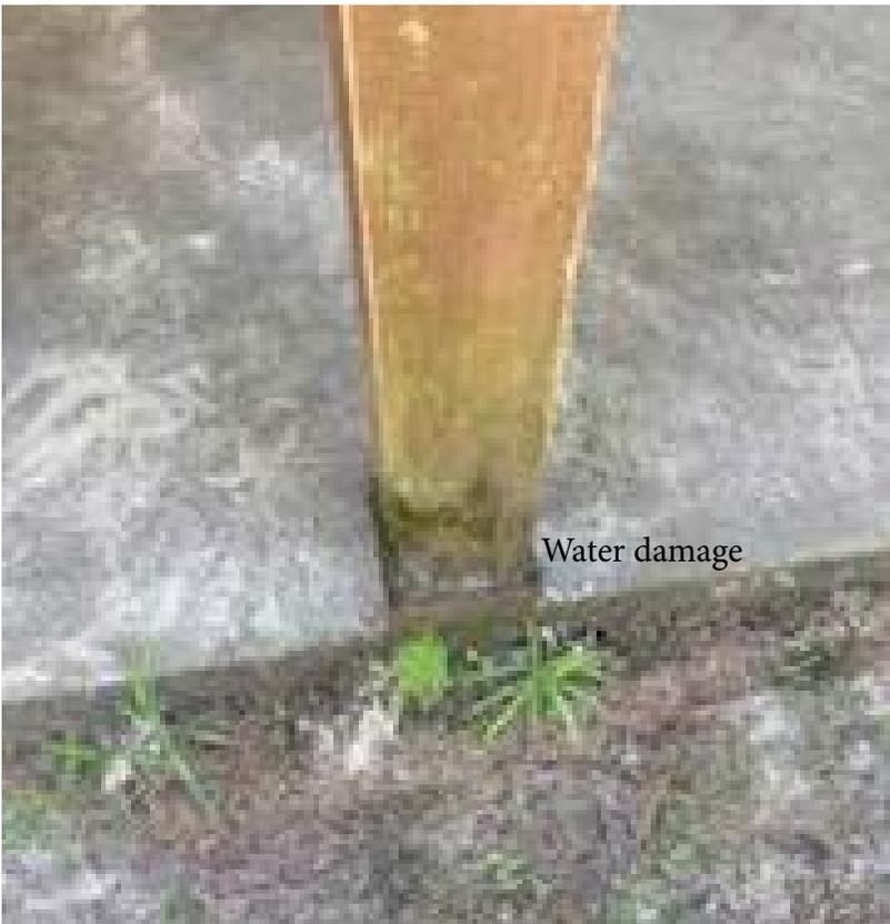
The restroom building at the swim beach has exceeded the expected lifespan. The structure will be raised to prevent water damage from to sea level rising and the intensity and frequency of storm events.
