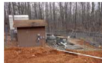
The old wastewater treatment plant was retired and removed.
