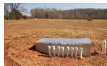
Old farm field for subsurface system was replanted, but trees aren't allowed.
